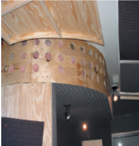
Figure 4: Unfinished Bass Trap above Recording Station
